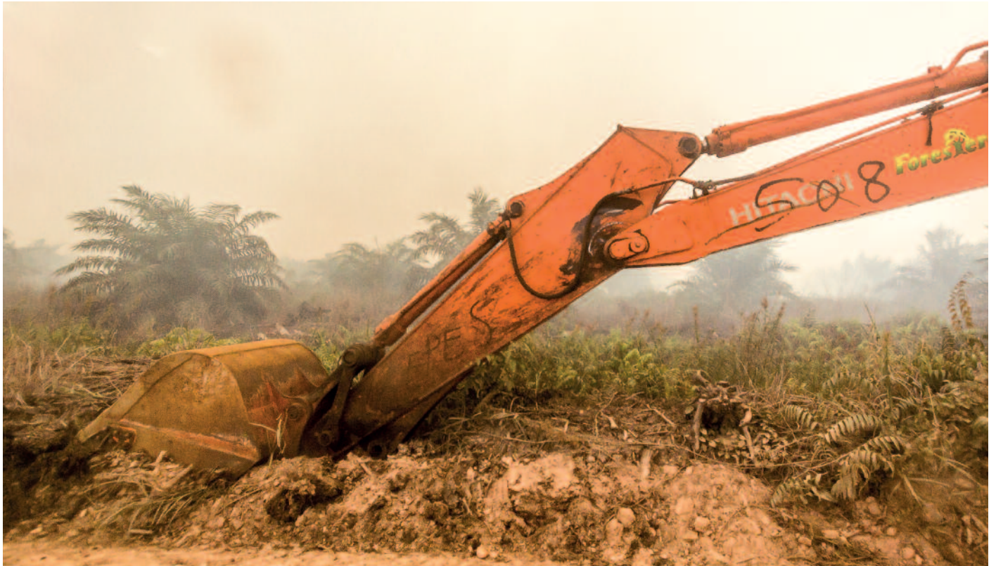
Excavator in BGA concession, Central Kalimantan, September 2015. © Victor Barro/FoE
