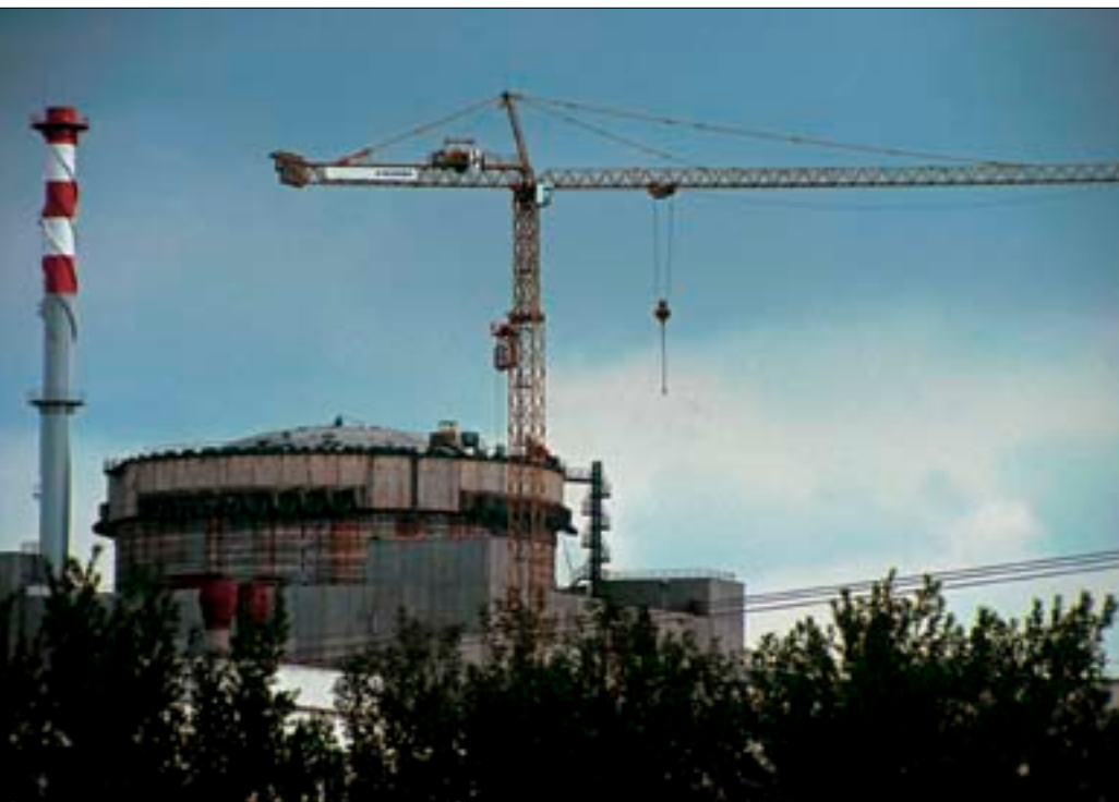
Construction work at Temelin nuclear power plant 1997.
